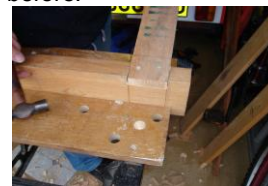
Picture 8 – Attach the legs with a couple of 5 cm nails.
